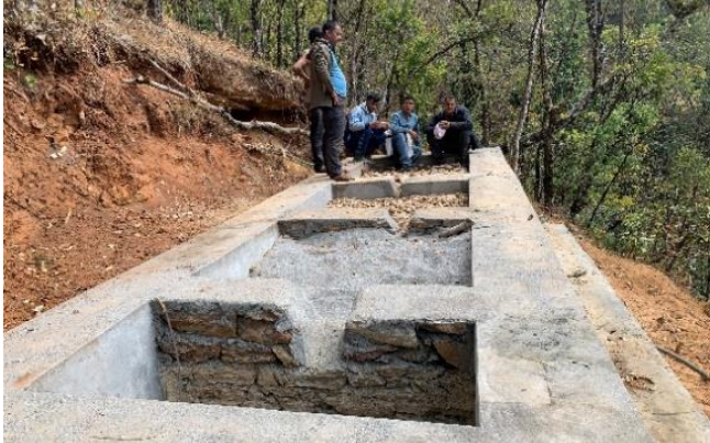
Photo 2: Horizontal roughing filter (©Keshav Kumar B.C.)
