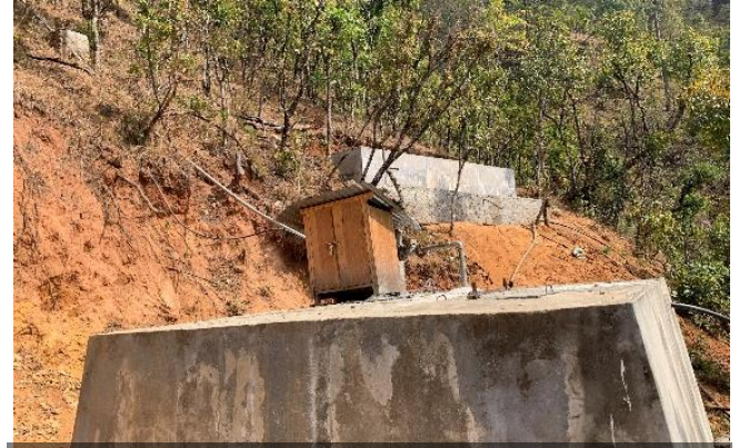
Photo 3: Water collection tank (©Keshav Kumar B.C.)
